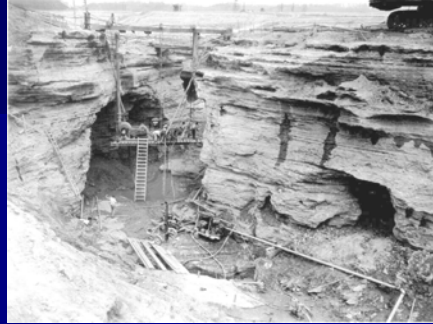
Caves along cutoff trench – Wolf Creek Dam
