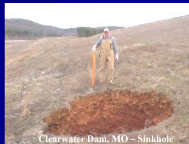
Clearwater Dam, MO – Sinkhole 15 January 2003
