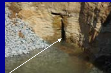
Open flowing 20 to 30 gpm under low head
