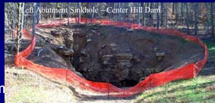
Left Abutment Sinkhole – Center Hill Dam
